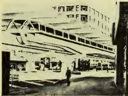
The nation's first commercial monorail will travel the 1.2 miles between downtown Seattle and the Fair in 95 seconds carrying 10,000 passengers per hour.
